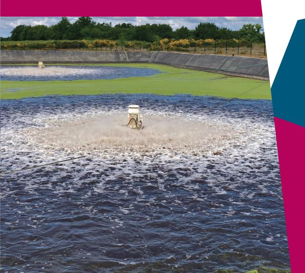
AERATION AND MIXING OF SHALLOW AND MEDIUM DEPTH TANKS, LAGOONS & PONDS
