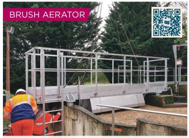
HORIZONTAL SURFACE AERATOR MANUFACTURED WITH BLADES
