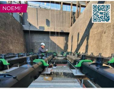
FIXED OR LIFTABLE FINE BUBBLE AIR DIFFUSER GRIDS
